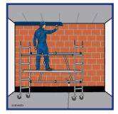
**Wall/ceiling connections** are easily and quickly sealed with Blowerproof brush or spray even on different types of material such as brick, concrete or steel. Different materials react differently to changes in humidity and temperature, which can lead to small cracks in plaster or other finishes leading to air leaks. Applied in two coats second coat must only be applied when the first coat has turned completely black.
