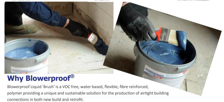
The water based polymer is brush applied to create an uninterrupted air and vapour-tight seals around penetrations, and for floor / wall connections, wall / ceiling joints, and roof connections.
