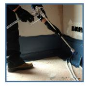
**Blowerproof Liquid Spray** A spray applied version, perfect for larger areas or direct application to insulation, masonry, brick and a wide range of substrates. Blowerproof Liquid Spray is the go-to solution for commercial and large projects where significant savings can be made due to its rapid rate of application. Blowerproof Liquid Spray is only available through approved applicators. Please call for more information or for a quote.
