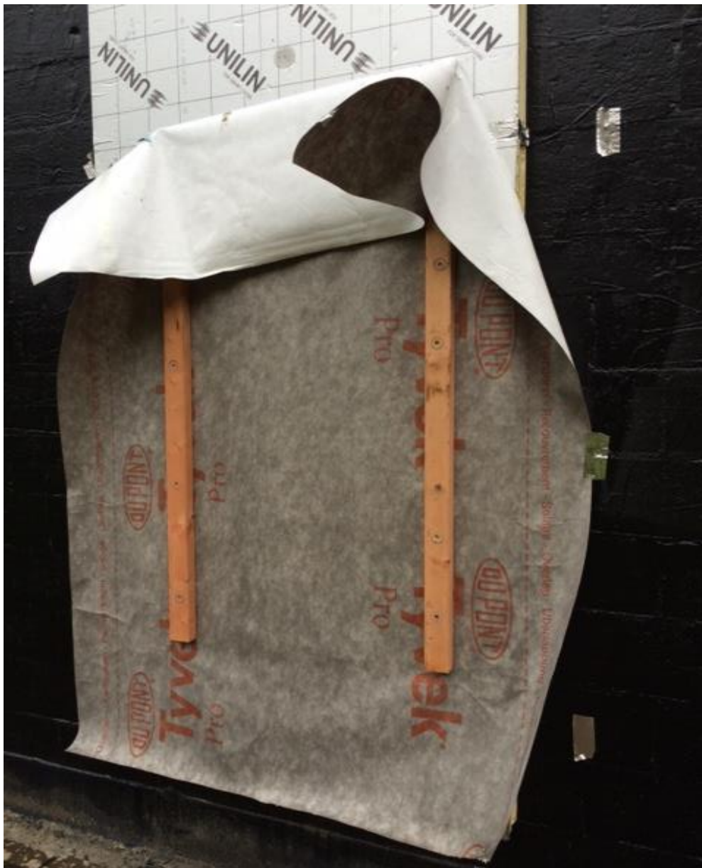
Photo 2/3: general view of perforations trough wall
